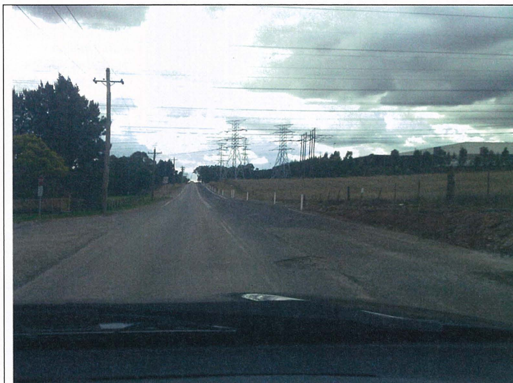
Photo of OWR showing pavement failure and potholing after widening works completed in 2011
